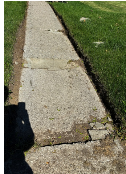
Current condition of walkway from street
